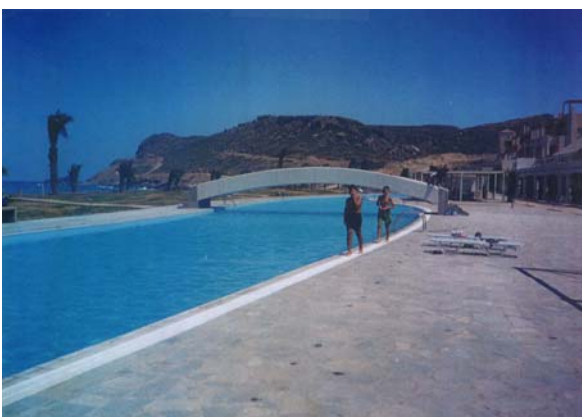
Dionysus Resort Housing Complex – Main Pool
