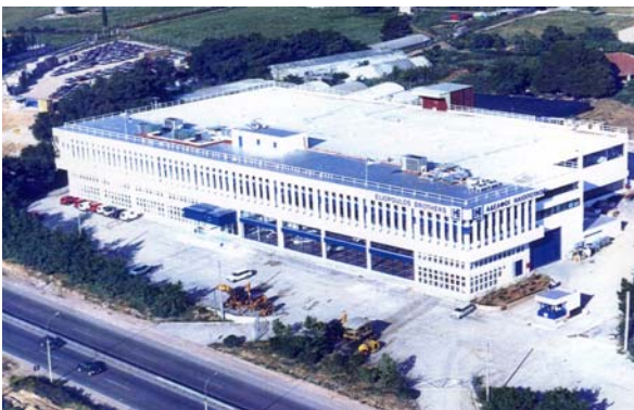
Office and Warehouse Building
