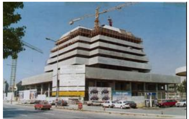
Onassis Cardiac Surgery Center (Under Construction )
