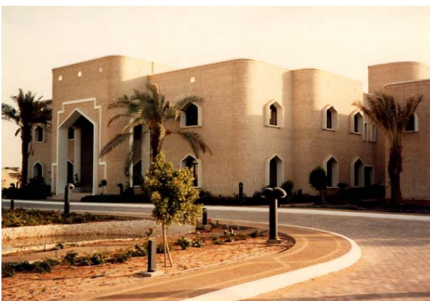
Sheikh Villa , Saudi Arabia – Façade
