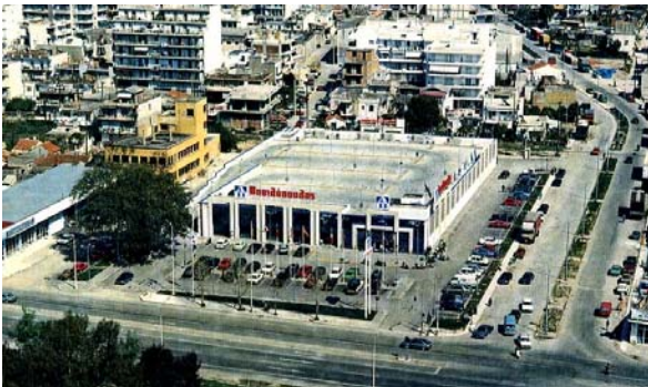
Supermarket Building, Patras
