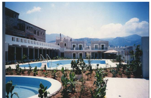
Dionysus Resort Housing Complex - Mall
